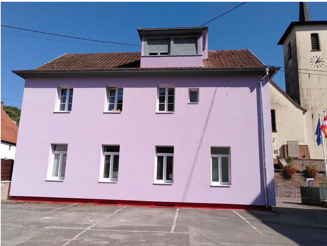
Figure 2. This picture shows the same school building after energy retrofitting. The traditional wooden shutters and decorative features of the façade have been removed, and the original stone
