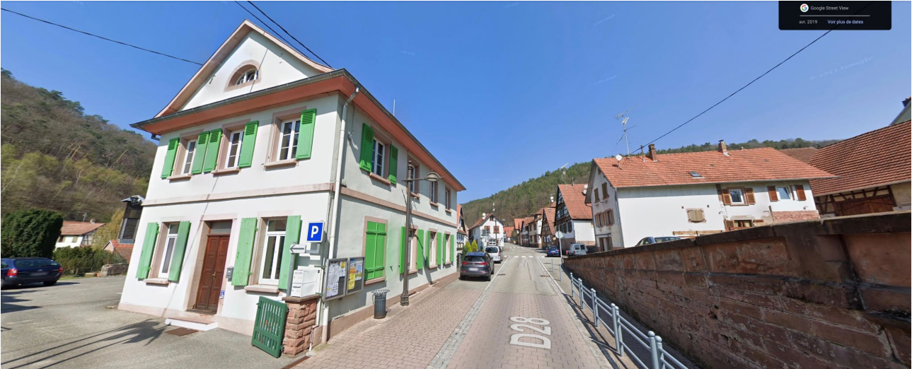
Figure 1. This image shows a school building in eastern France prior to energy retrofitting. Notable heritage elements such as traditional wooden shutters, original stone facades, and decorative features typical of the building's period of construction are clearly visible. These elements play a key role in preserving the historic character of the building and providing passive climate control by reducing solar heat gain.
